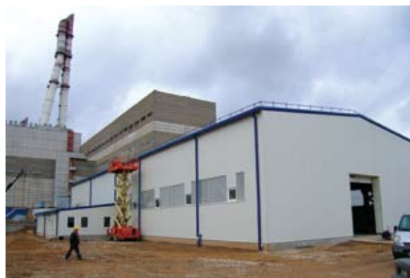
Picture 21. Ignalina NPP free-release facility construction finishing
