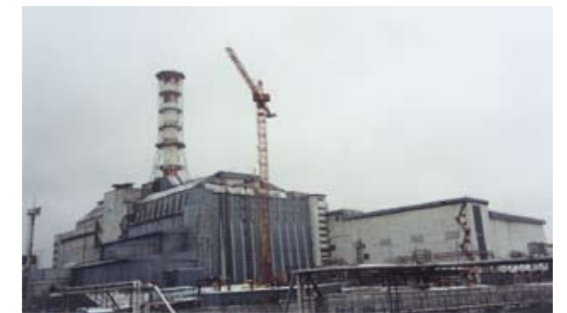
Picture 5. Chernobyl NPP Unit 3 Shelter.
