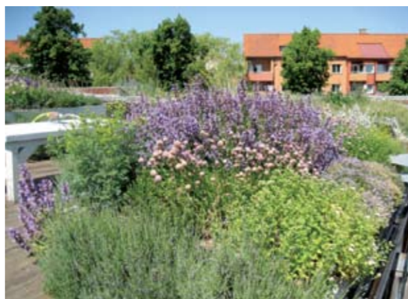
Picture 5. An intensive green roof, part of a recreational garden with wheel chair friendly floors Augustenborg, Malmö.
