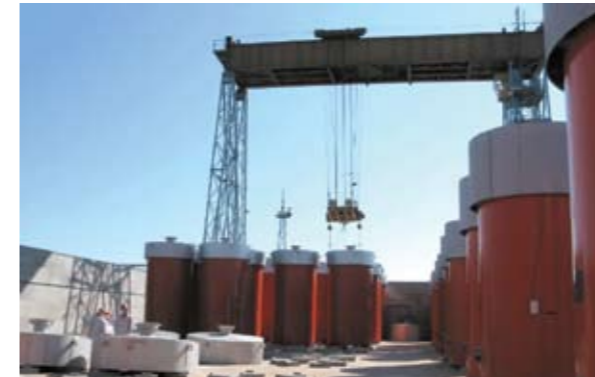
Picture 22. Ignalina NPP dry spent fuel storage
