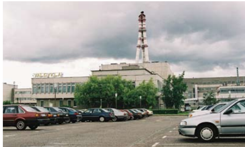
Ignalina Nuclear Power Plant, Lithuania
