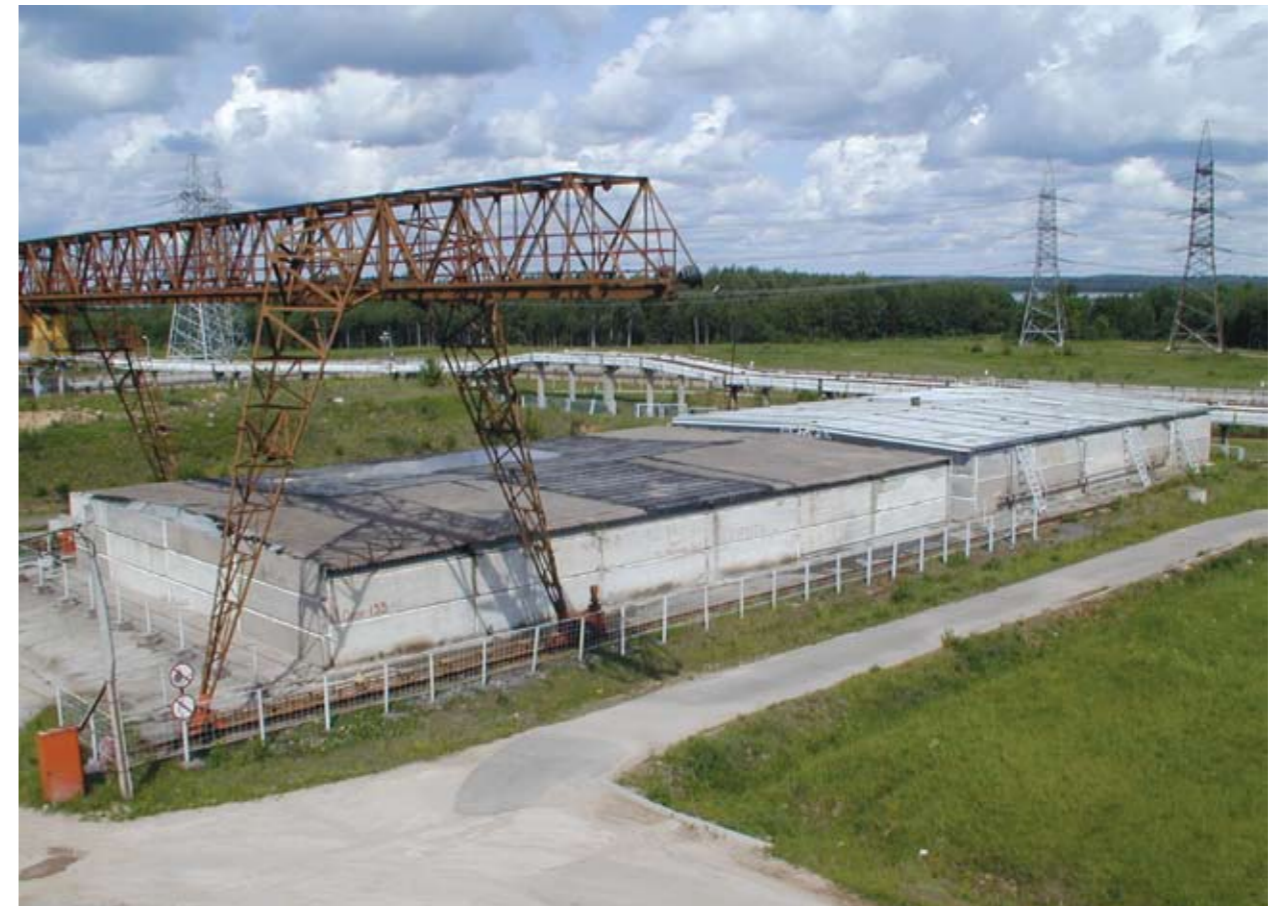
Picture 14. Ignalina NPP solid radioactive waste storage bunkers
