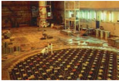
Ignalina RBMK reactor tube tops
