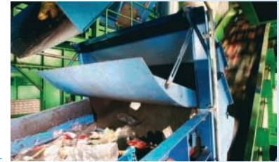
Air separator in action
