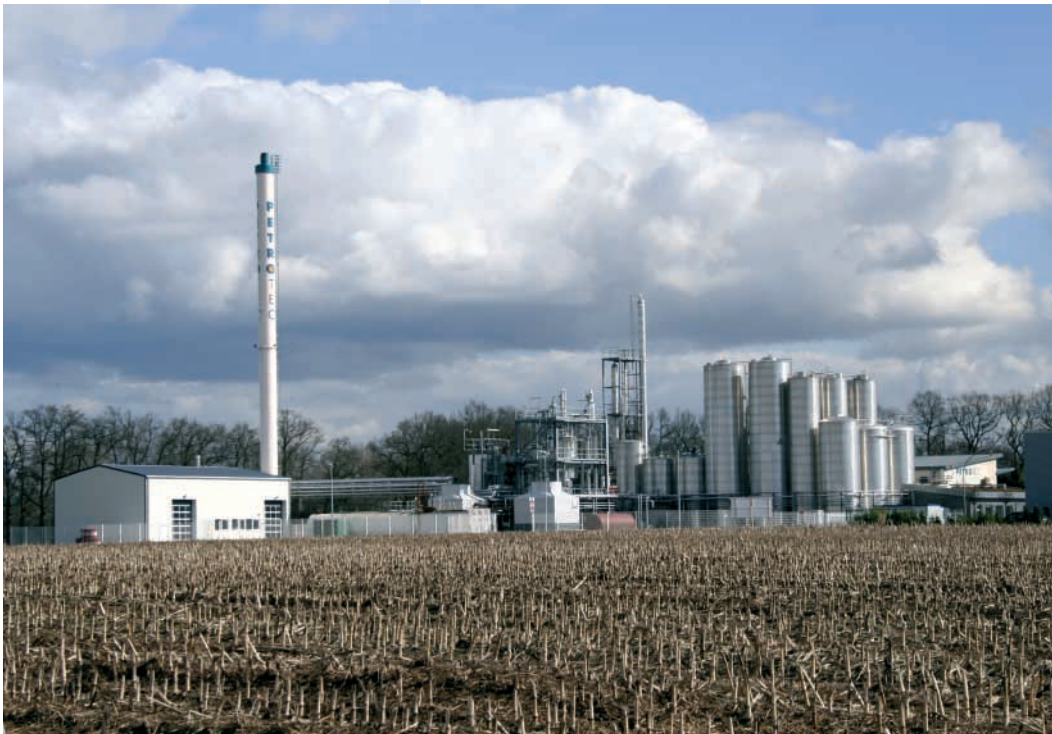
Fig. 5: Biodiesel Production Plant. State-of-the-art systems engineering makes a biogenous fuel out of waste fryer oil: methyl ester or "biodiesel" Source: PETROTEC GmbH, Borken
